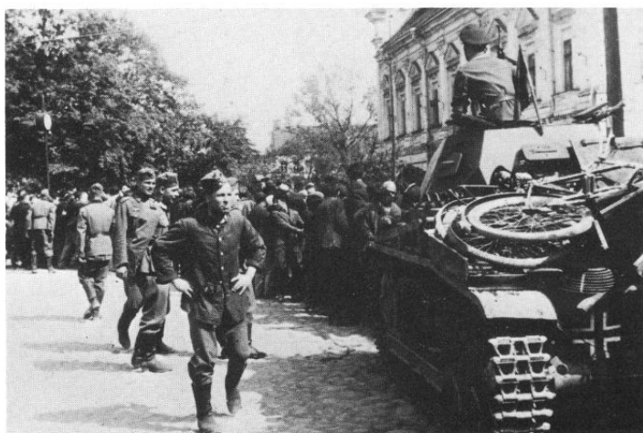
Another view of Jewish prisoners towing the broken down PzKpfw II Ausf. a. This shows the distinctive suspension, return rollers, driving sprocket and rear cooling air outlet of the old tank.
